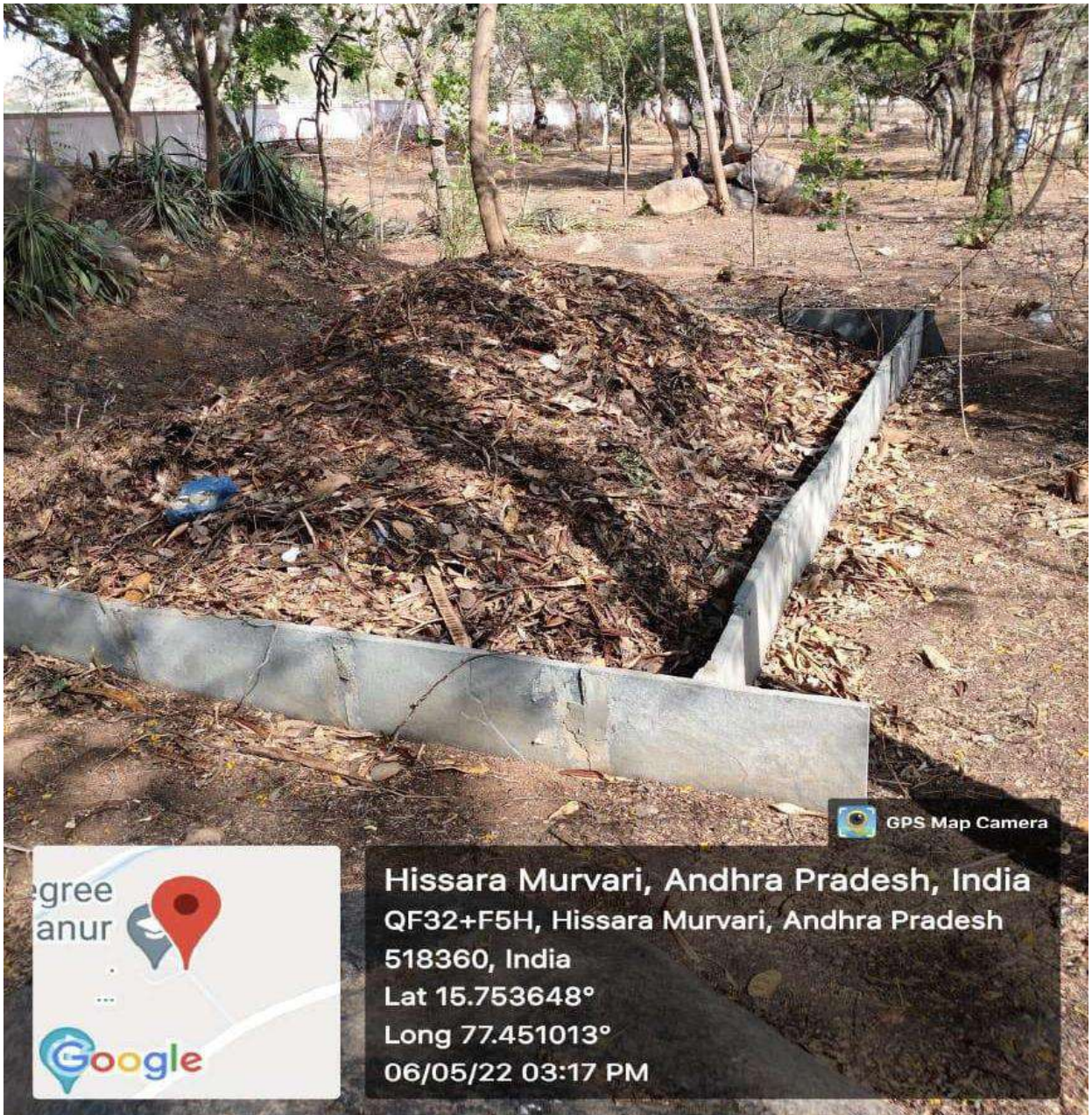
Degradable waste collection pit
